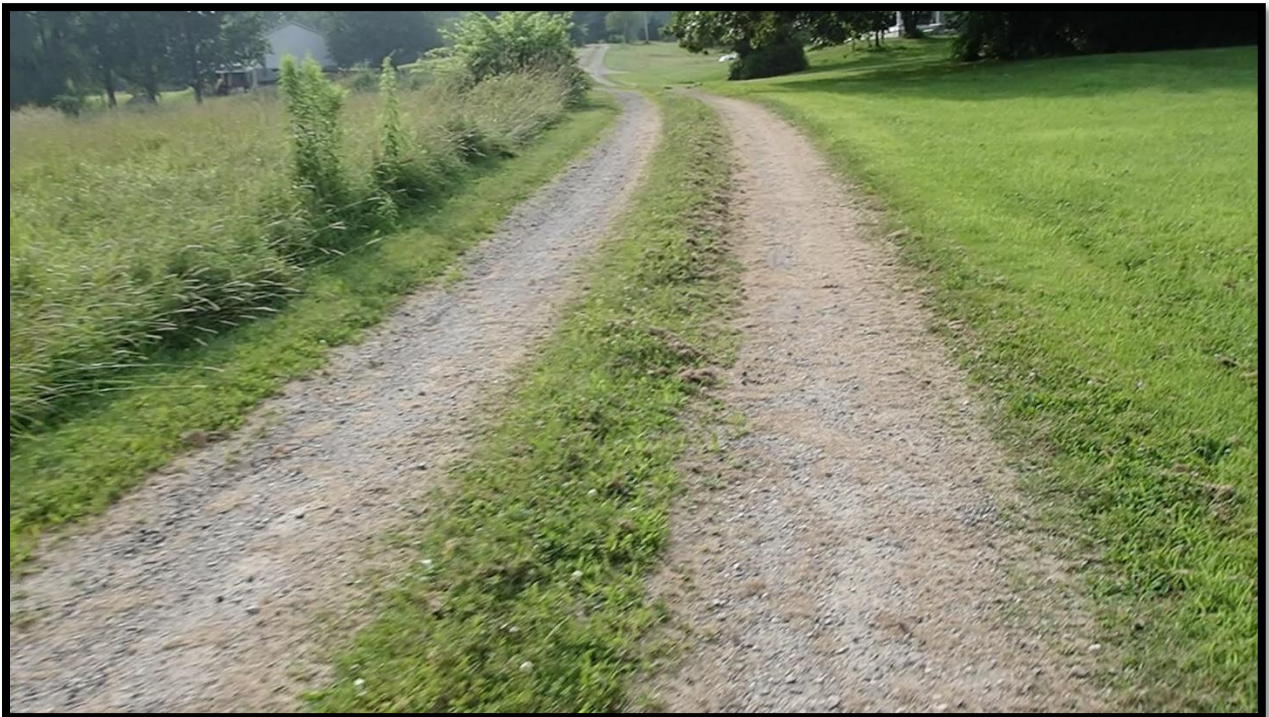
Photo 8. Facing West – Fitch Property in background
