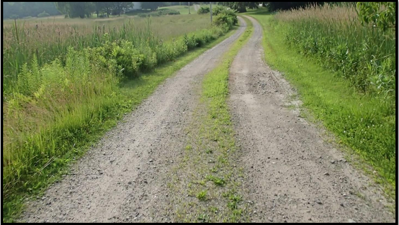
Photo 7. Facing West through wetland area, approximate location of (2) large diameter culverts
