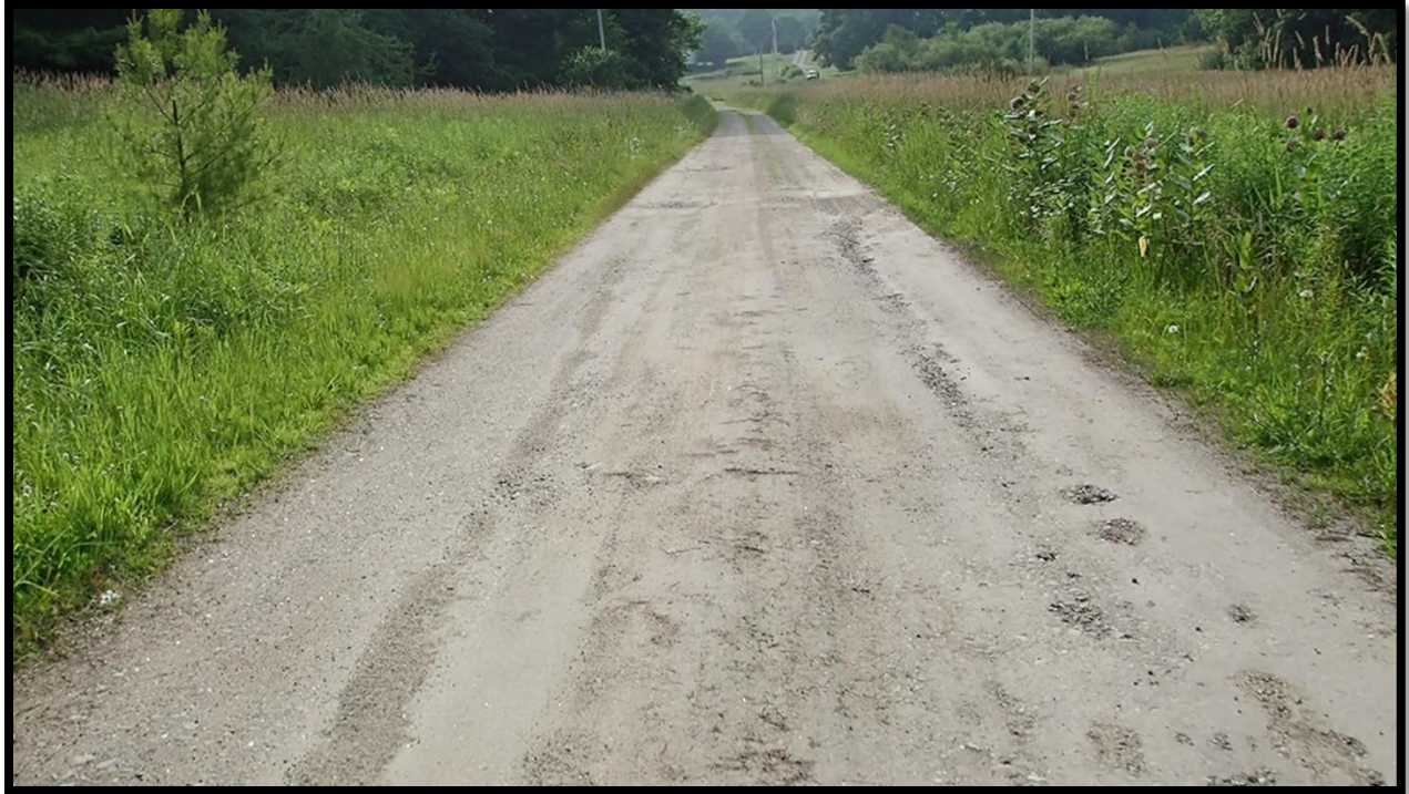
Photo 5. Facing West through wet meadow/Eversource ROW portion of driveway
